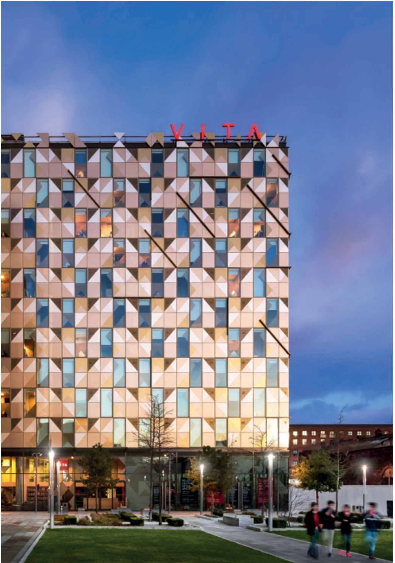
Manchester, First Street
