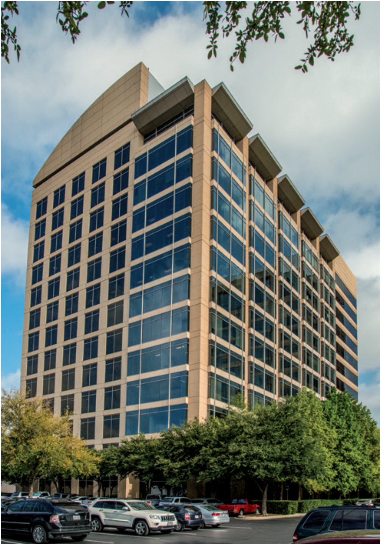
Dallas, Galleria North Tower II
