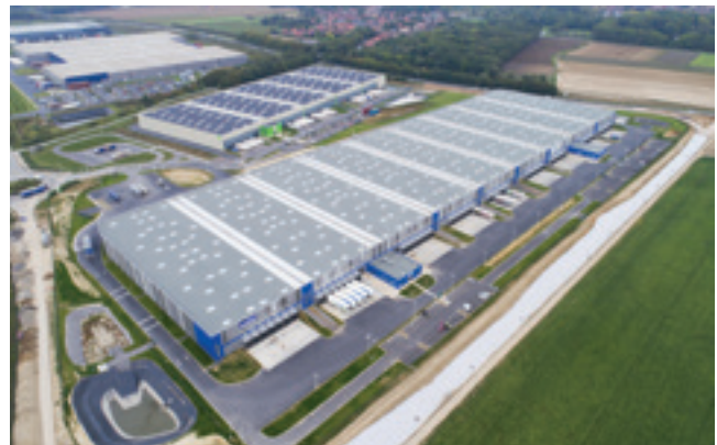
Lauwin-Planque Logistics Centre
