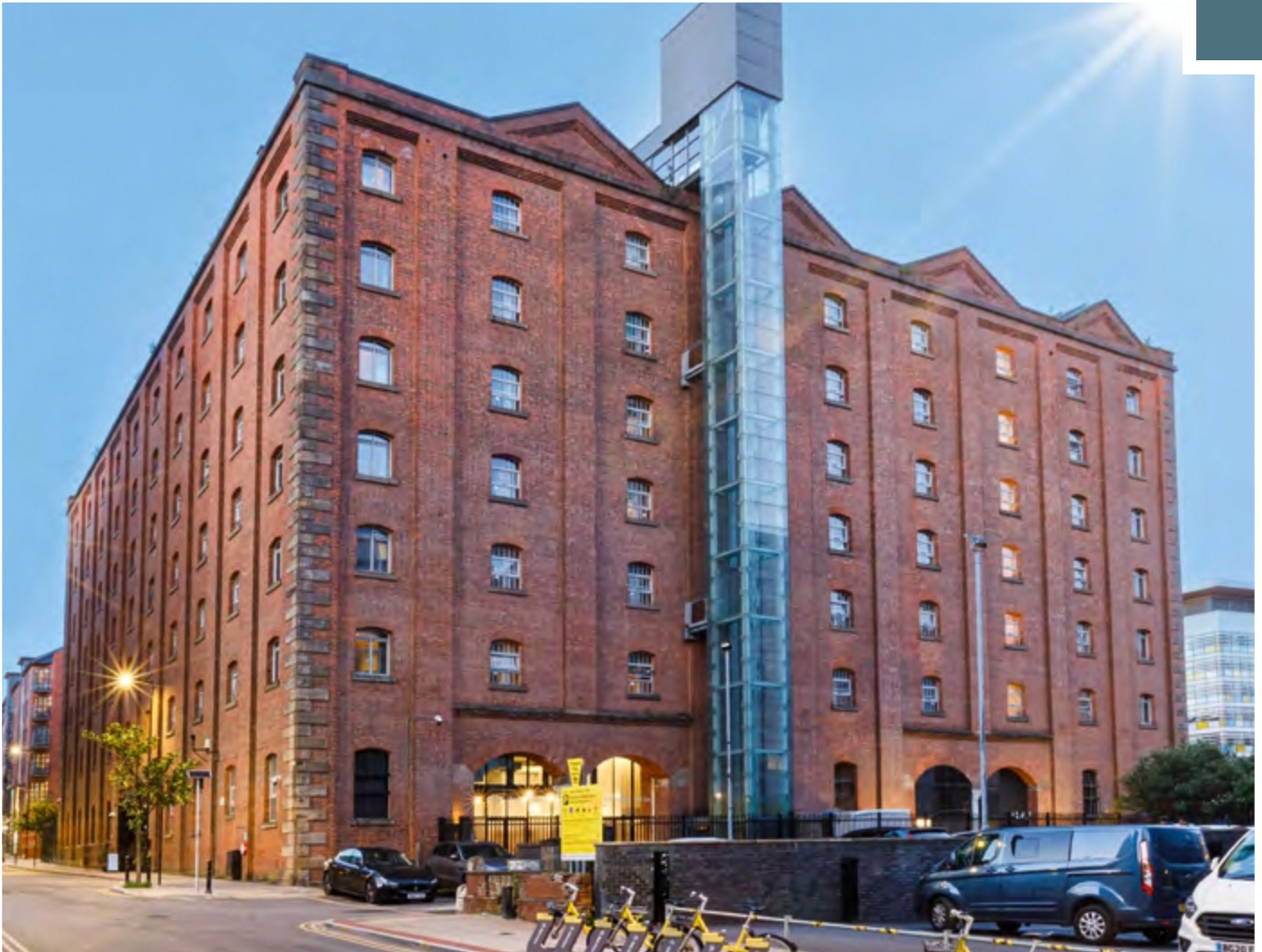
Manchester, 51 Ducie Street
